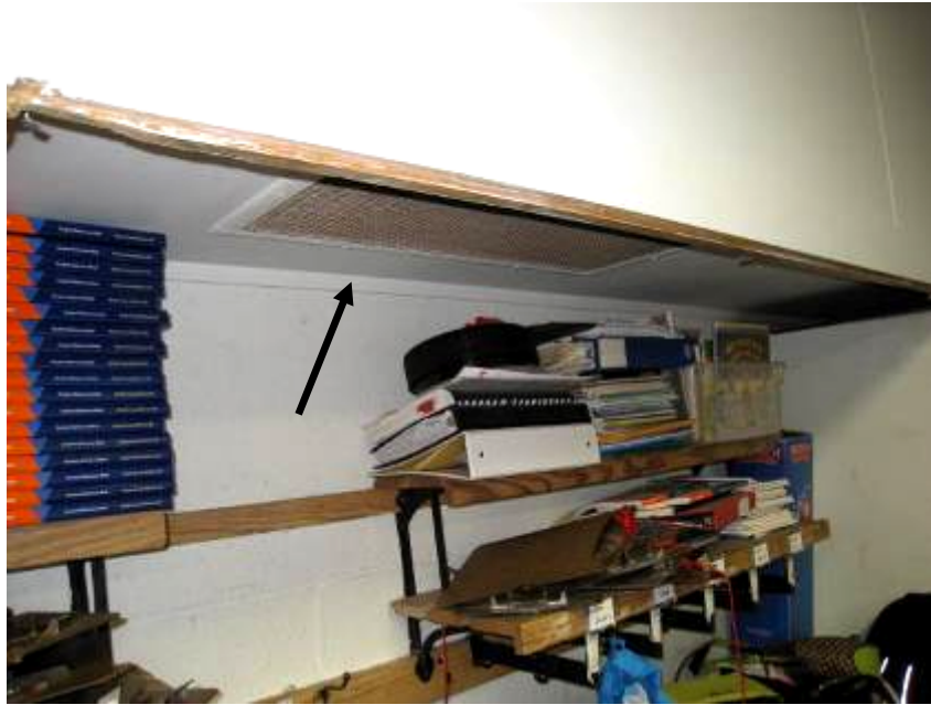
Exhaust Vent in Classroom Shelving
