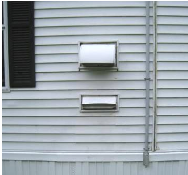
Air Intake Directly Above Exhaust Vent on Exterior Wall
