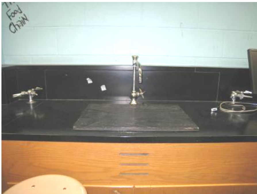
Covered/sealed science lab sink
