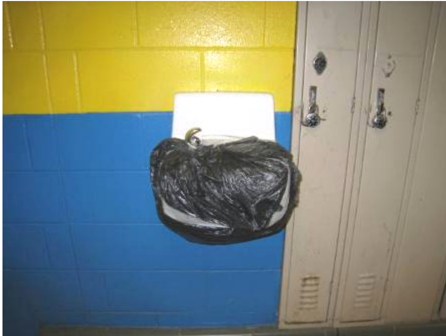
Out of service water fountain
