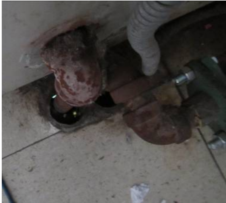
Pipe to univent cabinet with spaces (see light) around it to floor below
